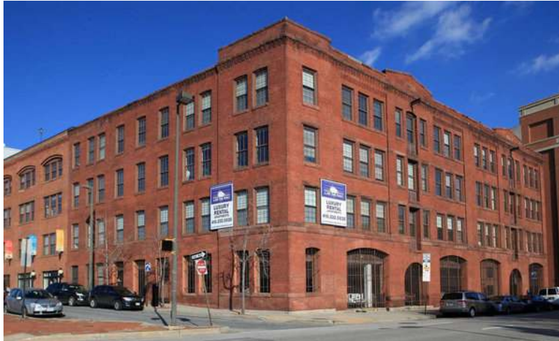
Daniel Kline and Delancey Street Capital recently bought the Sail Cloth Factory Apartments in Baltimore - $12.9 million for 107 units.
